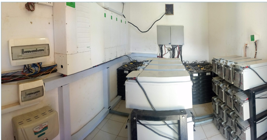
Installation of inverters, charge controllers and solar power system
