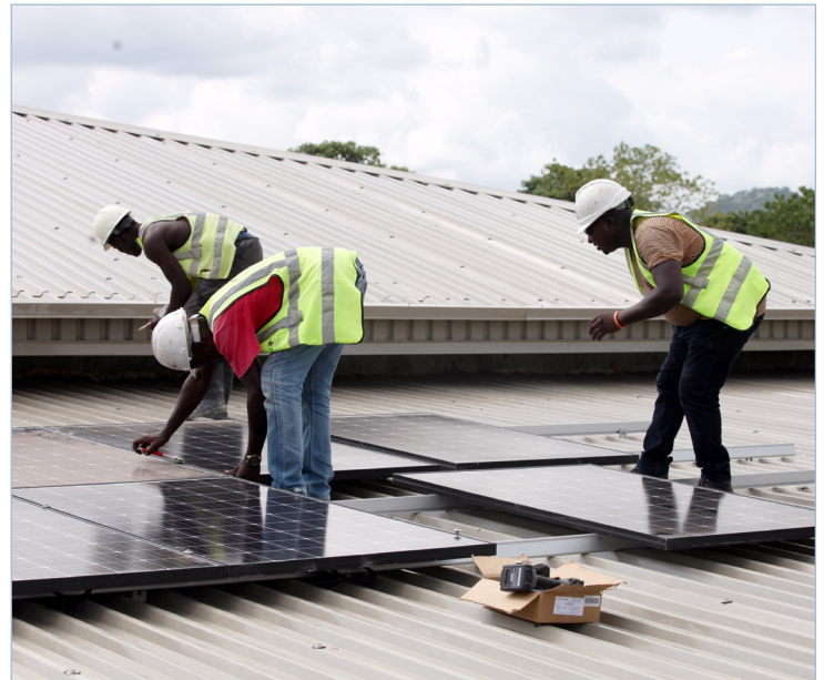
Installation of solar panels
